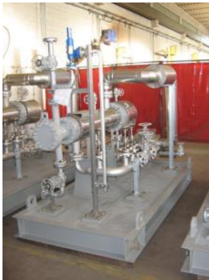
Nr. 4 Sealing Air Cooler Skid (insulated) 2,5 x 1,2 x 2,6 m – 1T GE OIL&GAS – Florence (Italy) for Saudi Aramco
