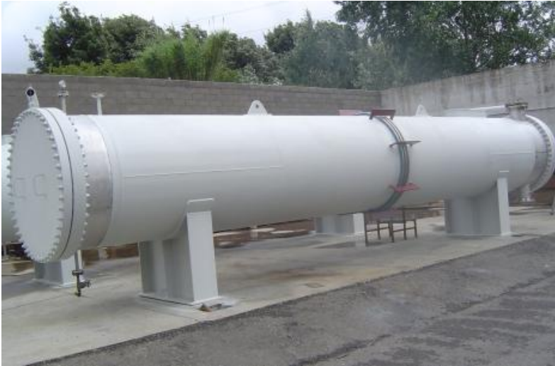
Nr. 6 alcohol production Heat Exchangers Ø 1,35 x 10 m AGRANA Bioethanol – Pischeldorf (Austria)
