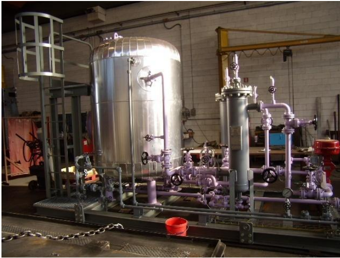
Amine Purifier Skid Busalla Plant (GE) PF10 - Milan (MI)
